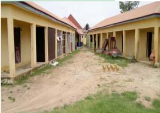
Admin Block – TIC Kaduna
