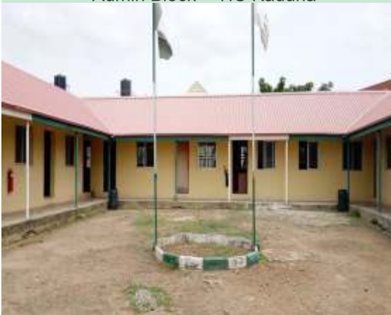
Admin Block – TIC Kaduna
